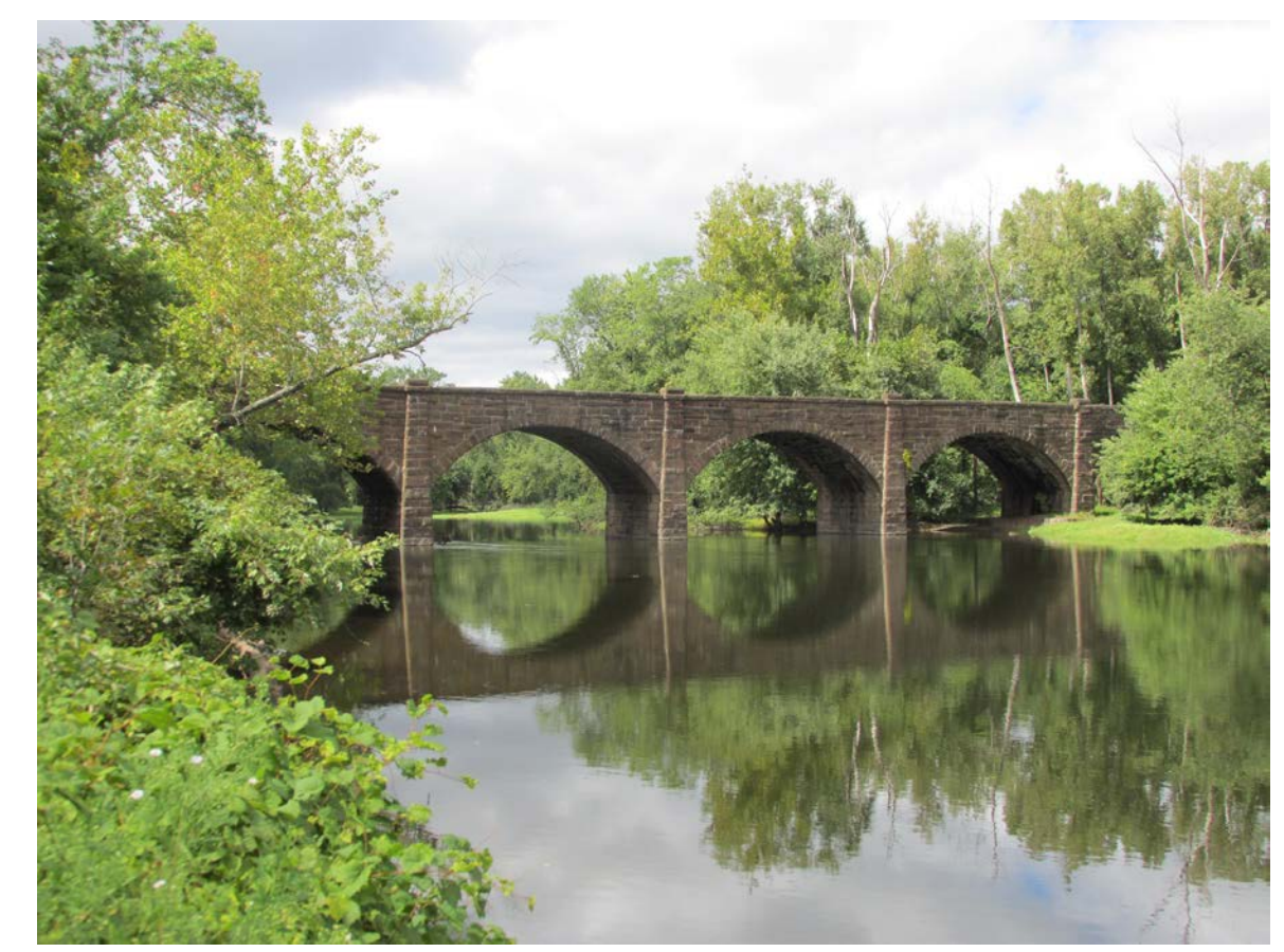
Farmington River Railroad Bridge
